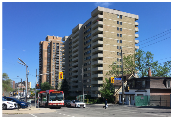
Large scale residential development
