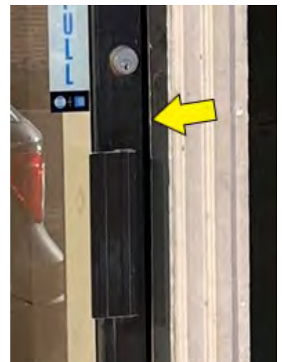
Note the large gap between the door and its frame (arrow). An astragal or, at minimum, a strike cover plate should cover the lock area.
