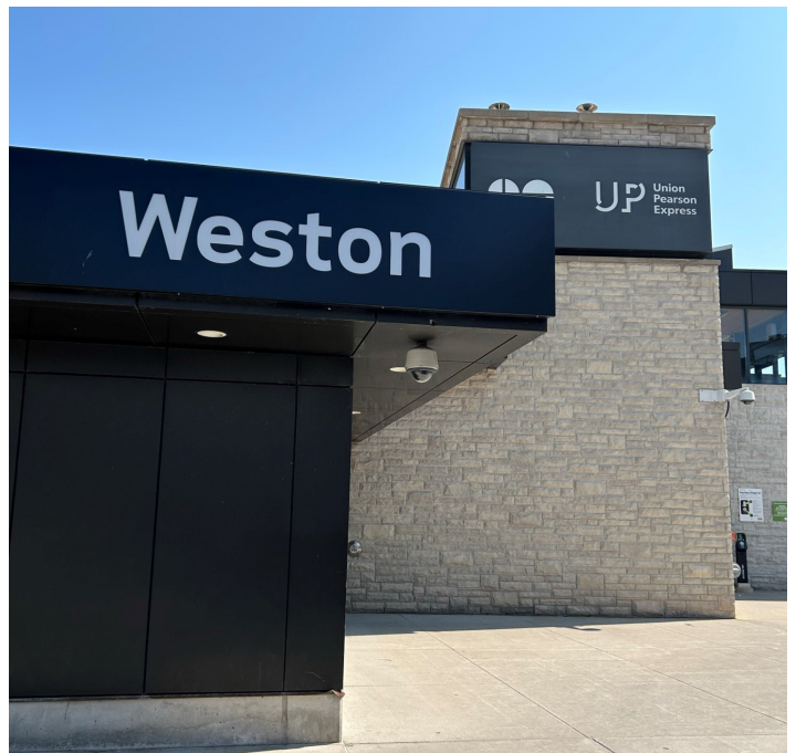
Figure 10 Weston Village GO/UP Station
